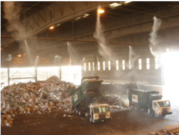
Photo: Benzaco Scientific A transfer station with its odor-control system in place
